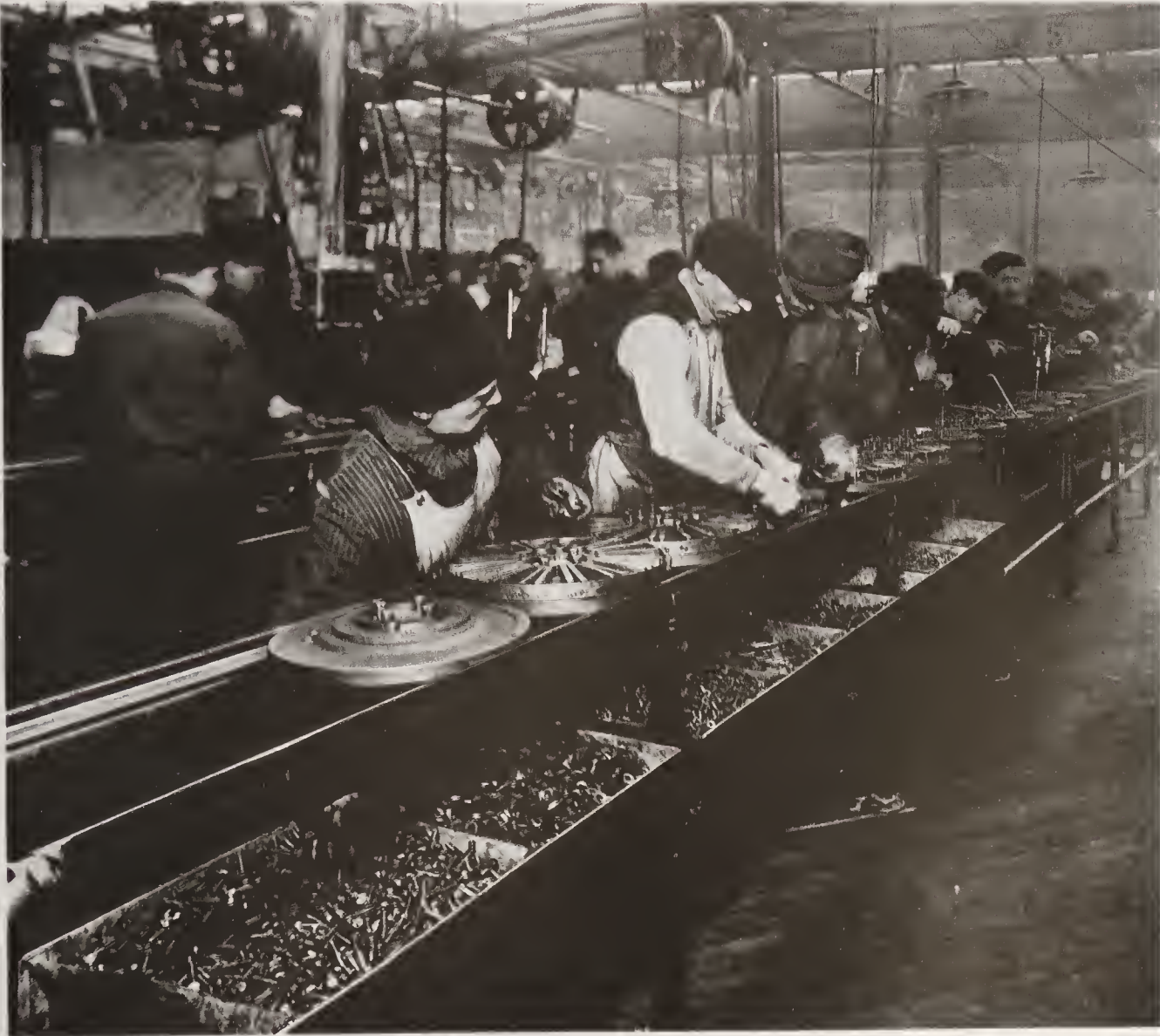
The magneto assembly line, introduced in 1913 at the Highland Park plant, was Ford's first assembly line.
