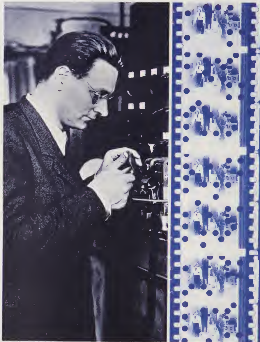
Zuse with the program reader of his Z4. Instructions for the machines were punched into discarded 35mm movie film.
