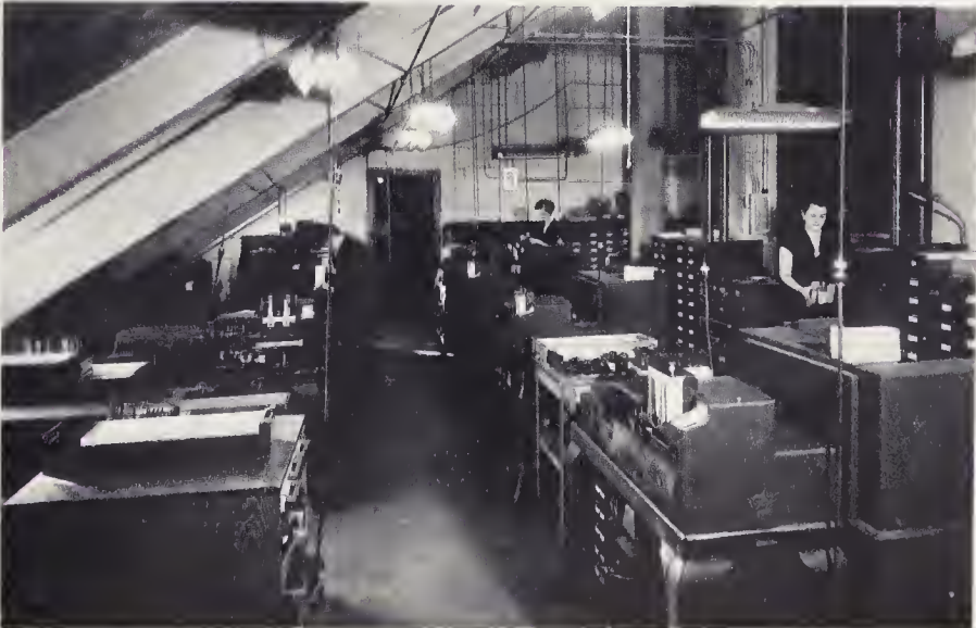
In 1940 Eckert left Columbia to become director of the Nautical Almanac Office. With war approaching, the immediate job was to produce quickly an Air Almanac for the Army's pilots. Eckert set up punch card machines to do the calculation and print out the results in a form that could be directly photo-offset.
